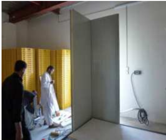
Technicians installing the sandwich panels of the cold room
