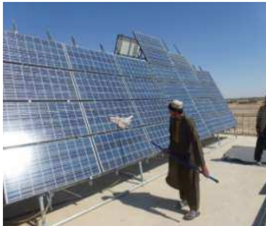
Solar panels (East side)
