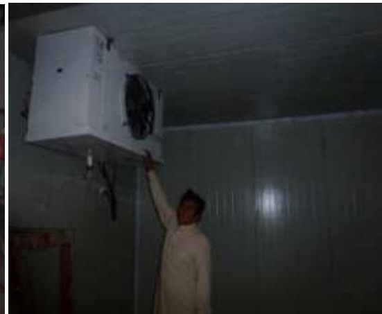
Evaporator installed
