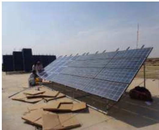
Solar panels being installed and cleaned (South side)
