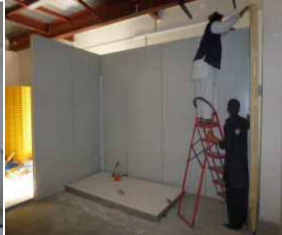
Technicians installing the sandwich panels of the cold room
