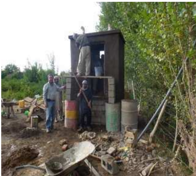
Latrine being built
